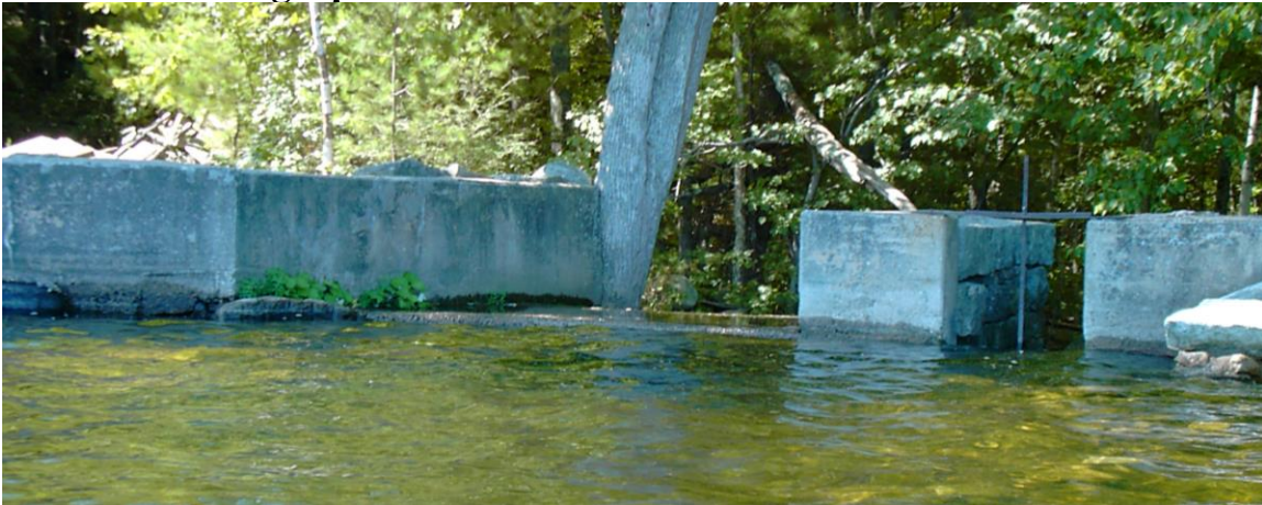
Dam Spillway and Sluiceway viewed from Keoka Lake
